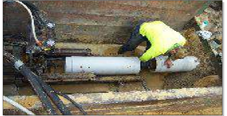
B250 installing 300 mm pipe
