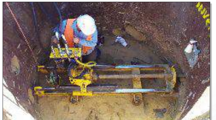
B110 pilot drilling for sewer
