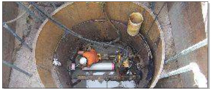
B750 at 7 m deep installing 225mm PVC sewer
